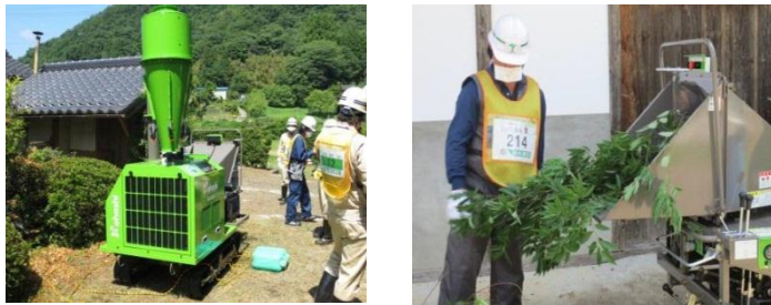
Chipping operation in decontamination site
