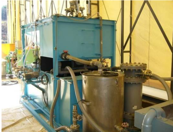
Water treatment equipment
