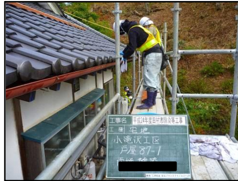
Wiping off a gutter
